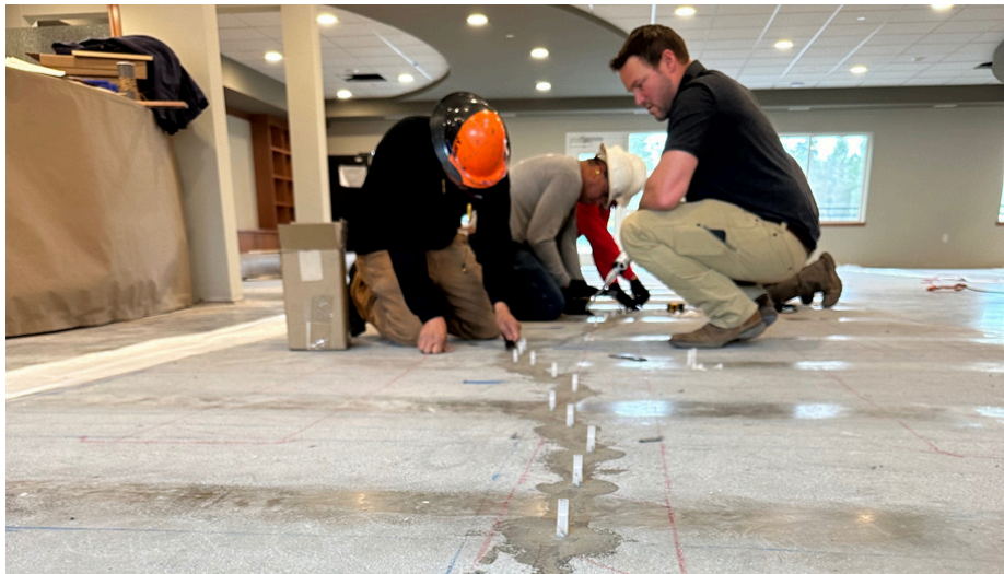
Due to gravity, the material flows downward and into the crack through the installed injection ports. The injection process is slow and controlled to ensure that the material fills the crack completely without creating air pockets, effectively bonding both sides of the broken slab together. Due to gravity, the material flows downward and into the crack through the installed injection ports. The injection process is slow and controlled to ensure that the material fills the crack completely without creating air pockets, effectively bonding both sides of the broken slab together.
