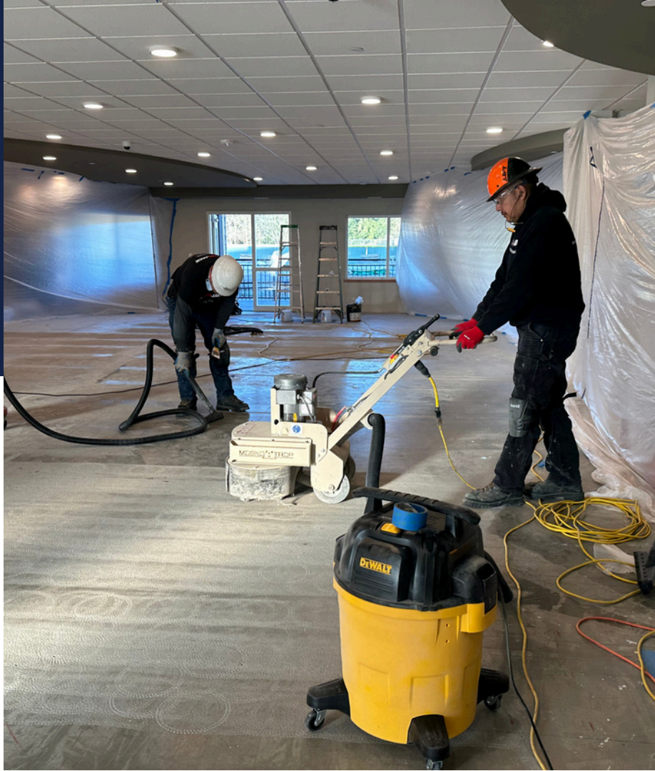
In this instance floor scarification was utilized to achieve the desired surface roughness of a CSP 4 on the top side of the slab. On the underside of the slab a diamond cup grinding wheel and dust extraction equipment was utilized to achieve a CSP 2. Bond testing was performed to confirm adequate results bonding to both the CSP-2 and CSP-4.
