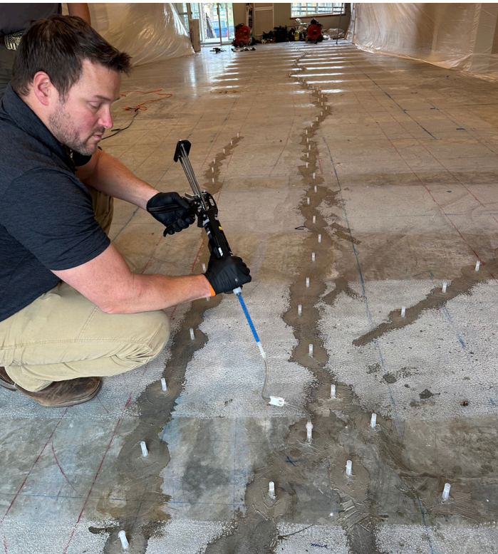
Due to gravity, the material flows downward and into the crack through the installed injection ports. The injection process is slow and controlled to ensure that the material fills the crack completely without creating air pockets, effectively bonding both sides of the broken slab together. Due to gravity, the material flows downward and into the crack through the installed injection ports. The injection process is slow and controlled to ensure that the material fills the crack completely without creating air pockets, effectively bonding both sides of the broken slab together.
