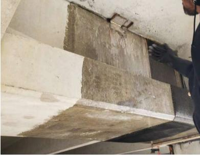
The project primarily involved the installation of Carbon Fiber Reinforcing Polymer (CFRP) on selected inverted T-beams to enhance structural reinforcement. This advanced material played a crucial role in strengthening support structures, ensuring stability, and improving load distribution.
