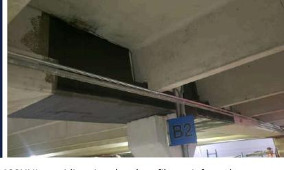
SRS worked with Bright Construction to get the SRS-600UNI, a unidirectional carbon fiber reinforced polymer (CFRP) approved for this installation. "U" wraps were specified for the inverted T-beams in order to repair and increase the shear capacity on the end spans of select beams where cracking was present. The addition of the CFRP, a surface applied, non-invasive, strengthening solution, is a great way to address damaged components and restore their structural capacity.
