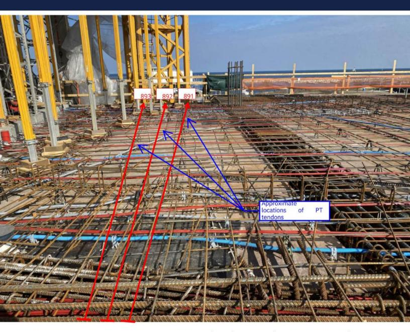
During an inspection on a recent high rise project it was discovered that three PT tendons were missed. Upon further investigation, it was found that without these cables, the slab did not meet the minimum requirements for temperature and shrinkage.
